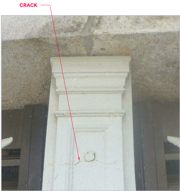
CRACKED CAST IRON PANEL WITH PIN
