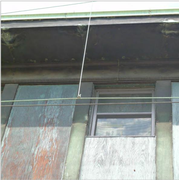
WATER STAINING, MISSING FASTENERS, BOARDED WINDOWS
