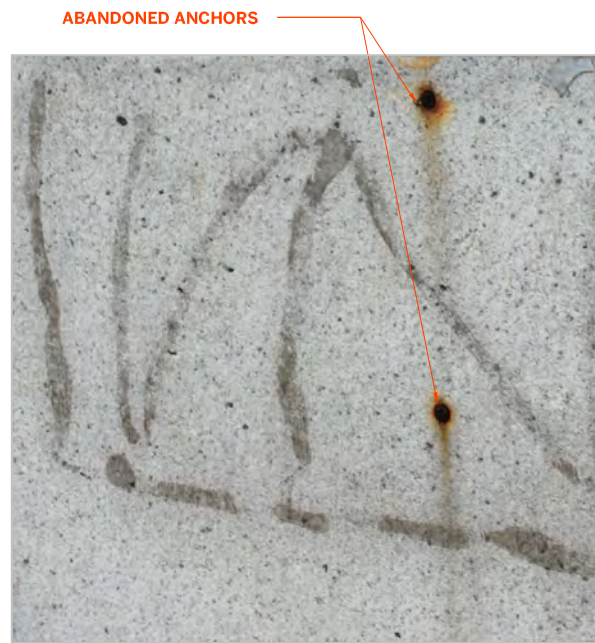
ABANDONED ANCHORS AND RESIDUE FROM FORMER SIGNAGE
