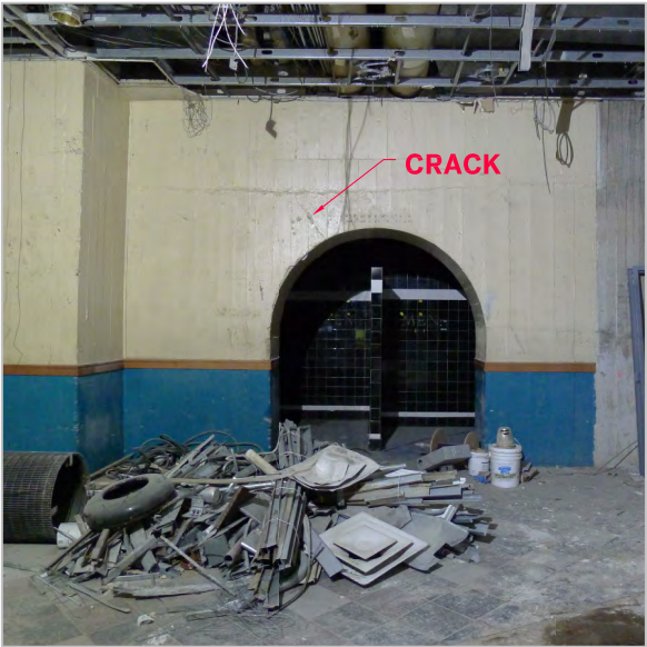
CRACK AT CONCRETE WALL
