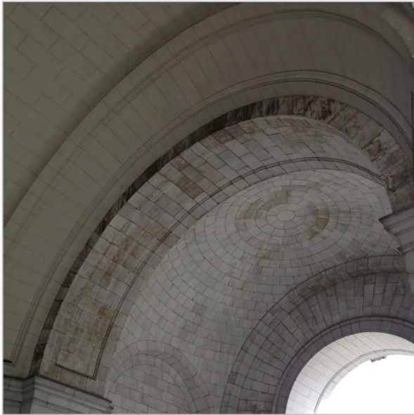
BIRD GUANO AND STAINING AT ARCH BETWEEN SOUTH PORTICO AND CARRIAGE PORCH
