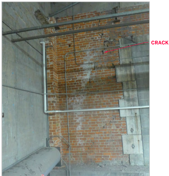
CONTINUOUS CRACK AT EXTERIOR WALL
