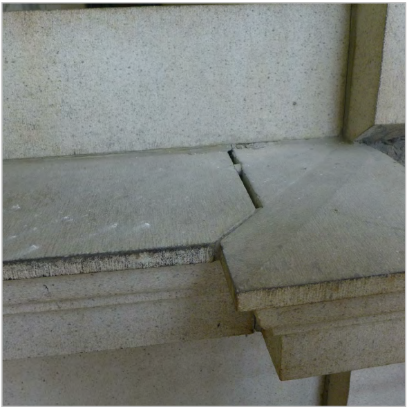
MORTAR LOSS
