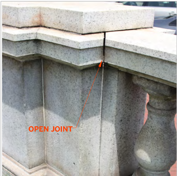
OPEN JOINTS IN BALUSTRADE ASSEMBLY
