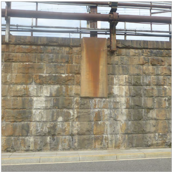
EFFLORESCENCE AND FERROUS STAINS
