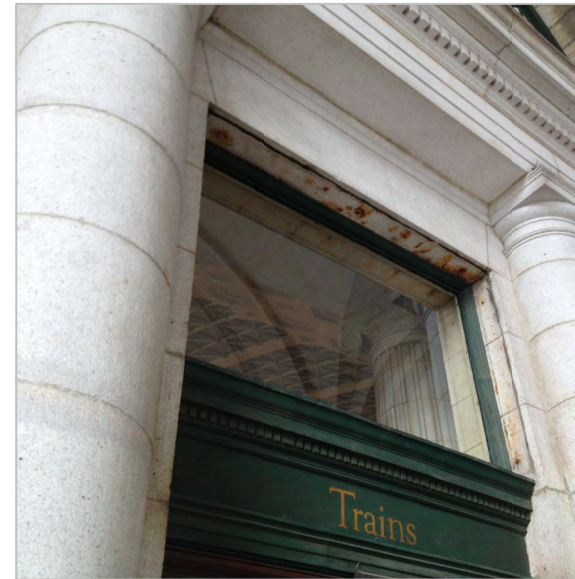
STAINING AND ABANDONED ANCHORS
