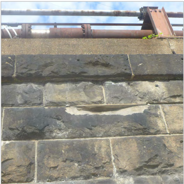
SPALLED STONE
