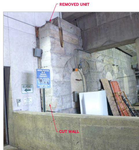
ORIGINAL MASONRY WALL CUT AT NEW RAMP
