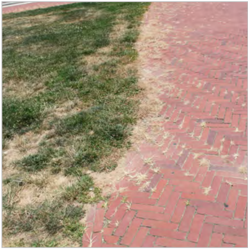
TURF GROWING OVER AN AREA OF DEPRESSED BRICKS
