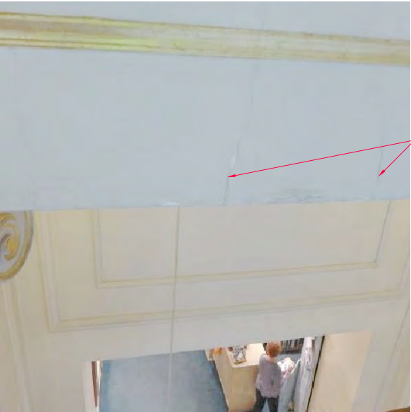
CRACK AT PLASTER SOFFIT
