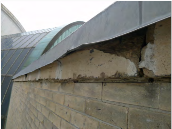
SPALLED TERRA COTTA AND BRICK
