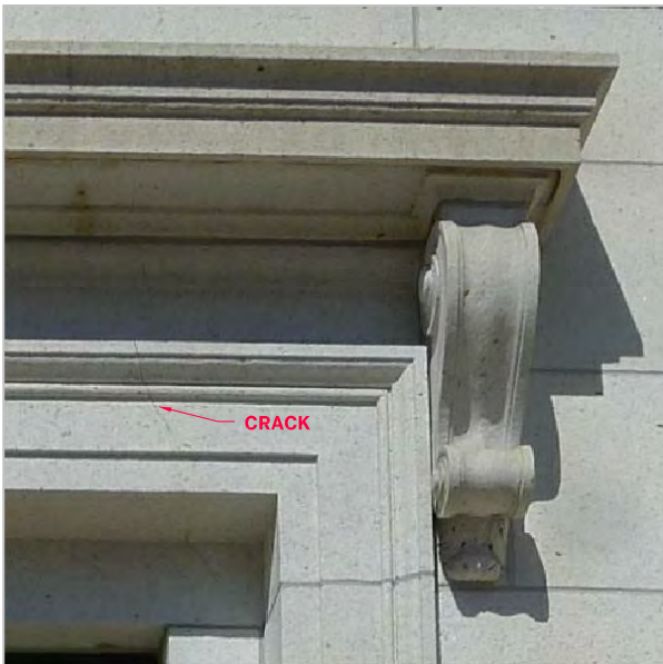
CRACK IN GRANITE WINDOW LINTEL
