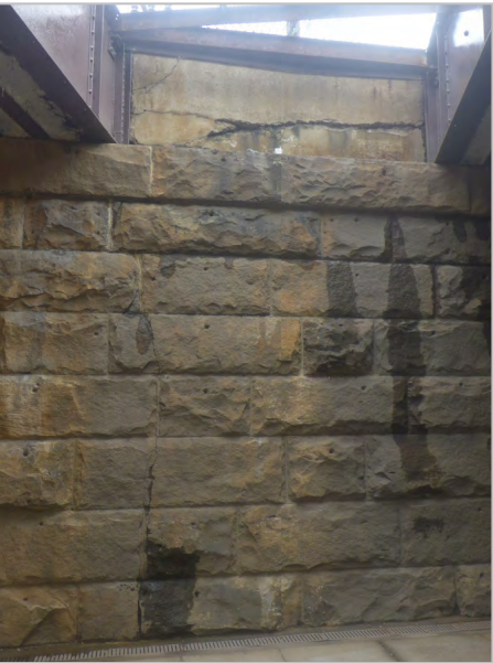
CRACKED STONE AND CONCRETE WALL AT M STREET UNDERPASS
