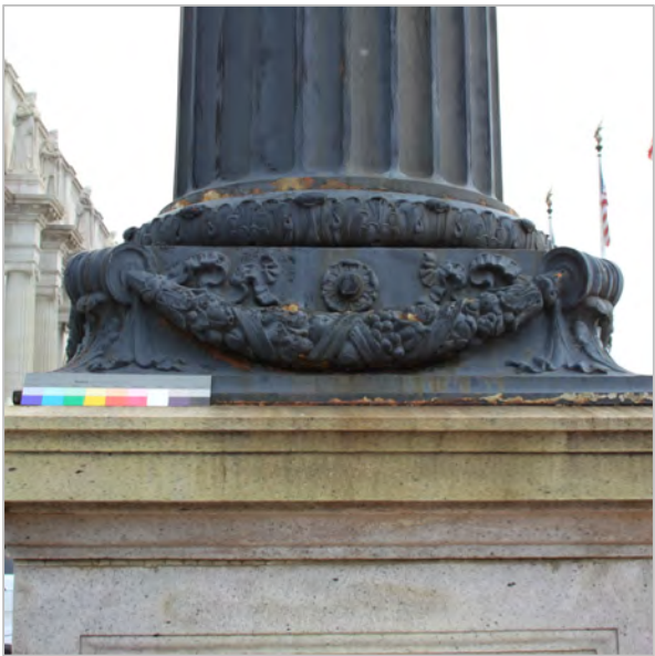
SURFACE CORROSION AND FERROUS STAINING ON GRANITE BASE
