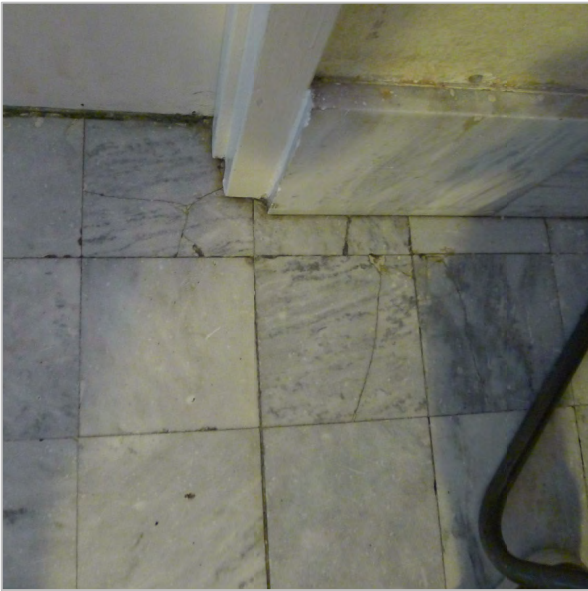
CRACKS AT MARBLE FLOOR TILES
