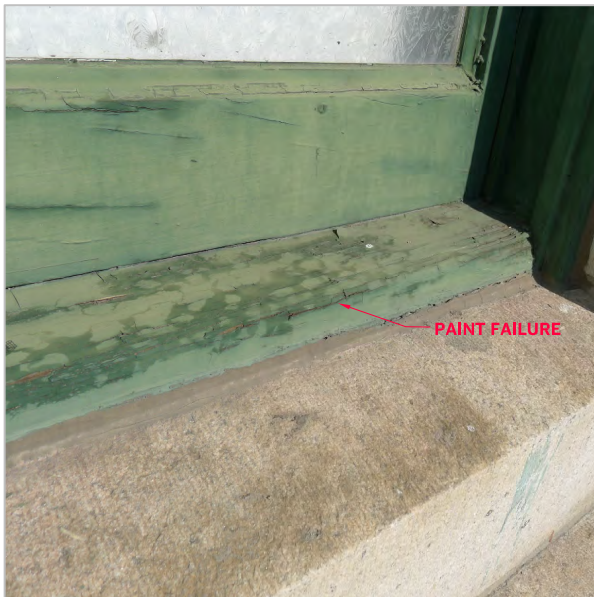
PAINT FAILURE AND DETERIORATED SEALANT AT WOOD WINDOW
