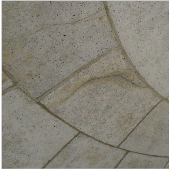
CRACK IN TERRA COTTA CEILING TILE
