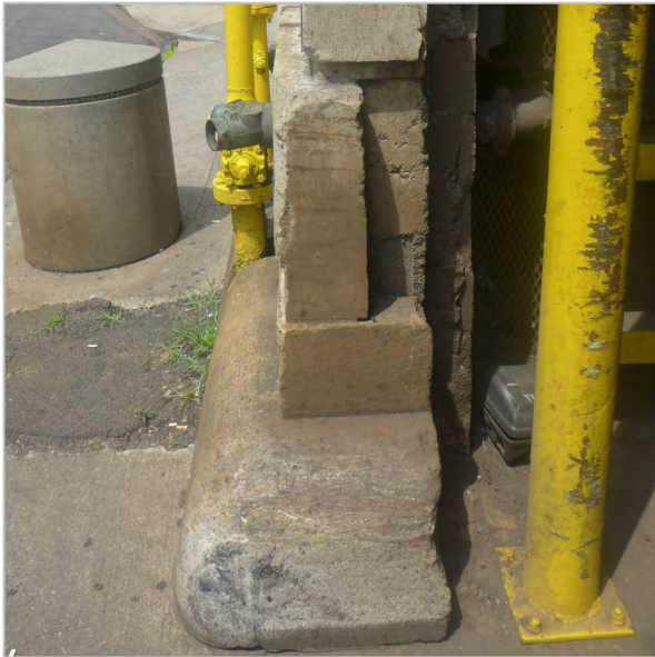
DAMAGED GRANITE JAMB
