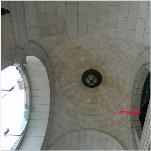
STAINING AT CEILING
