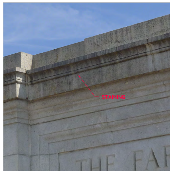
WATER INFILTRATION AND STAINING AT COPING STONES
