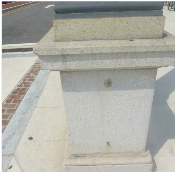
PATCHED HOLES AT GRANITE
