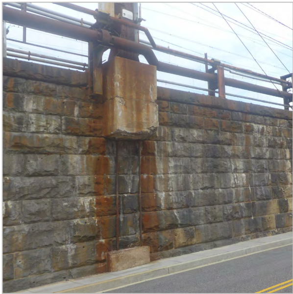
DETERIORATED AND CRACKED CONCRETE, EXPOSED REBAR AND FERROUS STAIN
