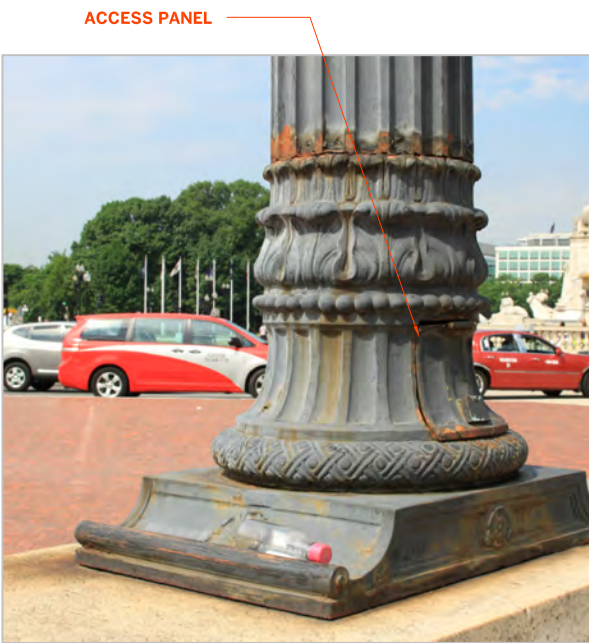
PAINT FAILURE AND CORROSION
