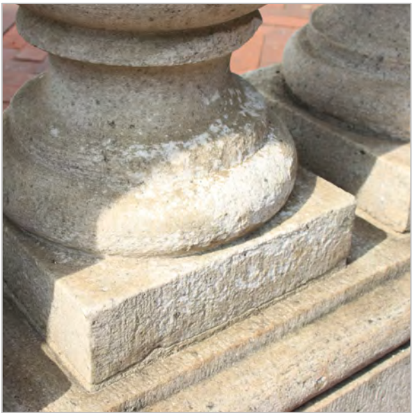
DISAGGREGATION OF GRANITE BASE OF BALUSTER
