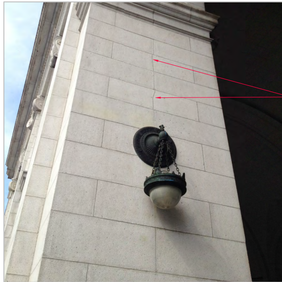
CONTINUOUS CRACK ABOVE LIGHT FIXTURE
