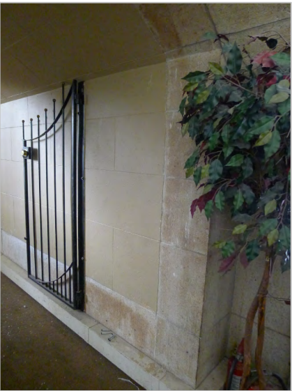
PAINTED GRANITE AND SOILING AT SOUTH GALLERY
