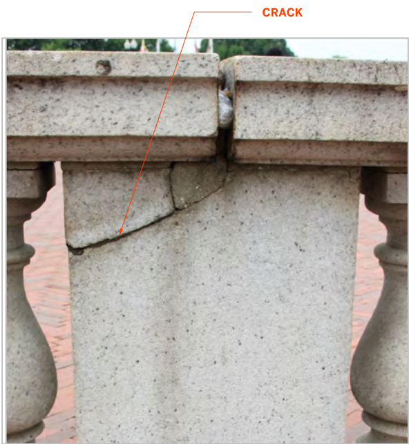
CRACKING THROUGH MASONRY
