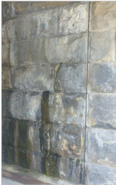
CONTINUOUS CRACK AT M STREET UNDERPASS
