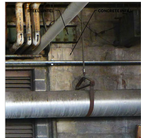
NON-ORIGINAL STEEL LINTEL AND CONCRETE INFILL
