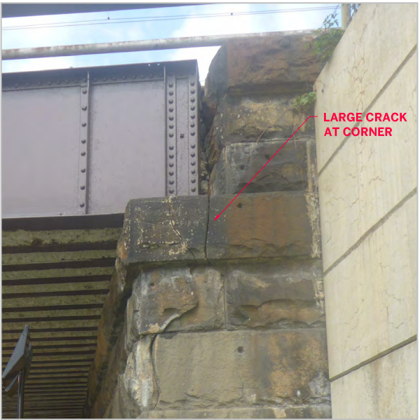
CRACKED CORNER STONE
