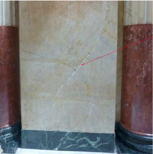
CRACKED AND LOOSE SCAGLIOLA PILASTER
