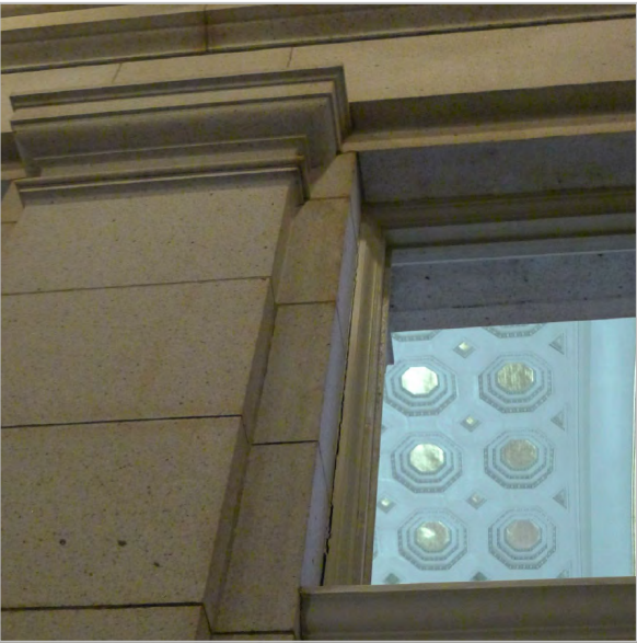
OPEN JOINT BETWEEN GRANITE AND FRAME
