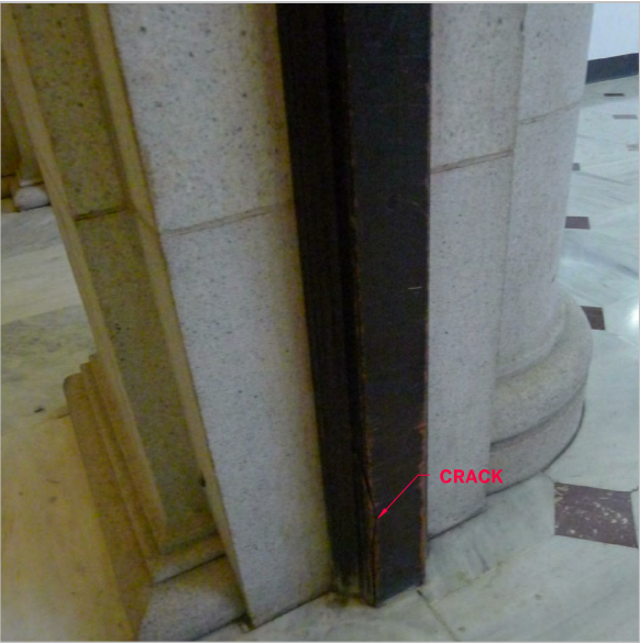
CRACK AT WOOD FRAME
