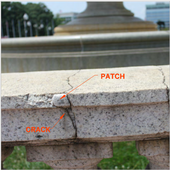
CRACKING AND PATCH THROUGH BALUSTRADE RAILING
