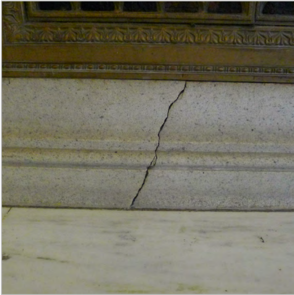
CRACK AT GRANITE BASE
