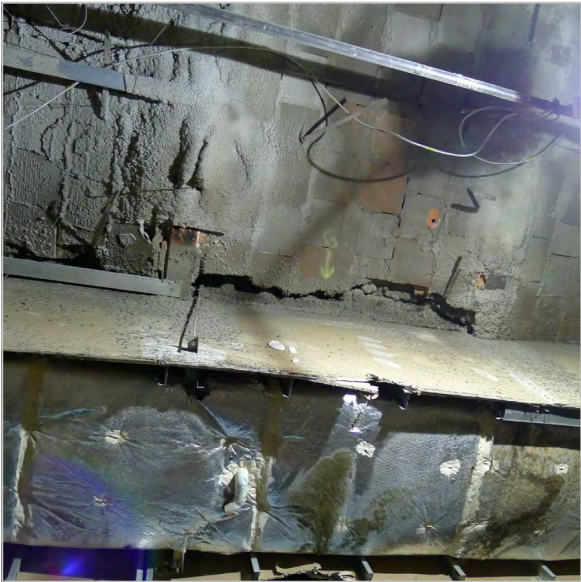
CRACKED TERRA COTTA SLAB
