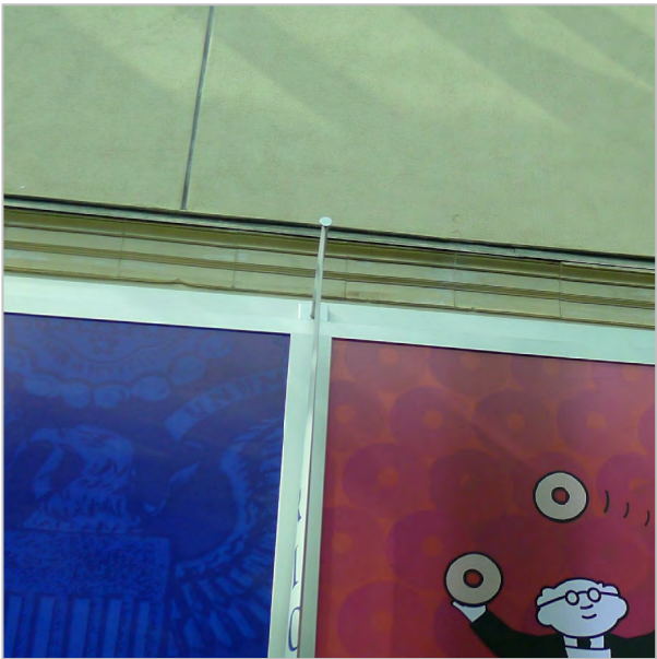
SPALLS AT TERRA COTTA CORNICE (FORMER NORTH EXTERIOR WALL)
