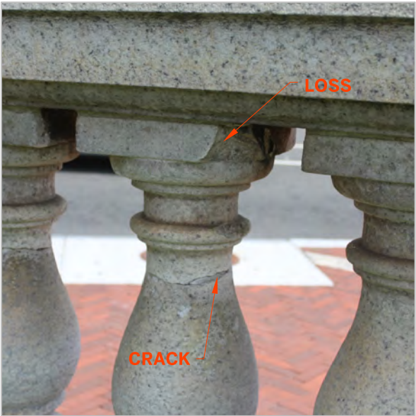
CRACKING AND LOSS AT BALUSTER
