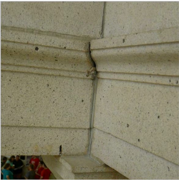
CRACKED AND OPEN JOINT
