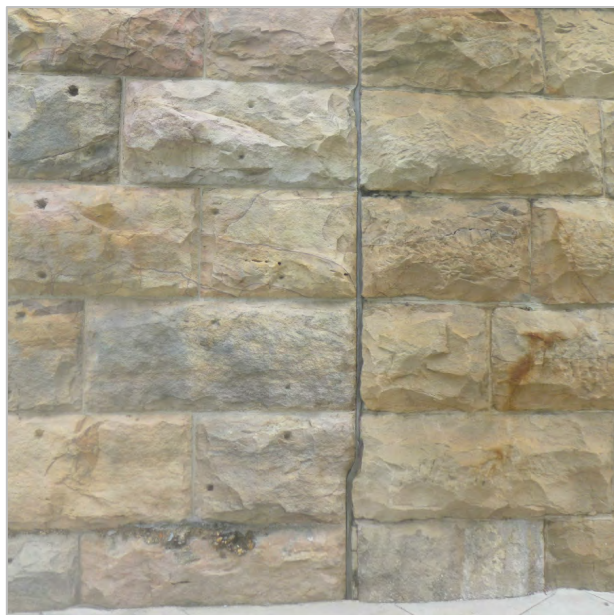
EXPANSION JOINT BETWEEN ORIGINAL AND REBUILT WALLS
