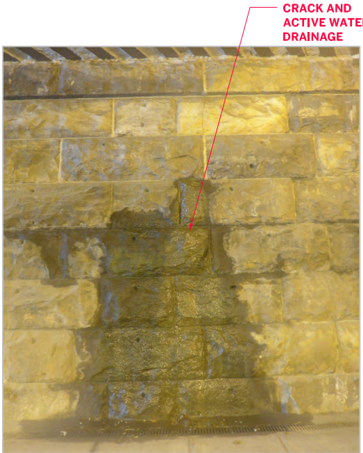
CONTINUOUS CRACK AT K STREET UNDERPASS
