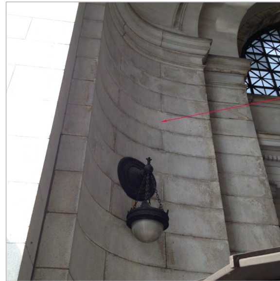
EVIDENCE OF WATER INFILTRATION, SURFACE LOSS AND SCALING
