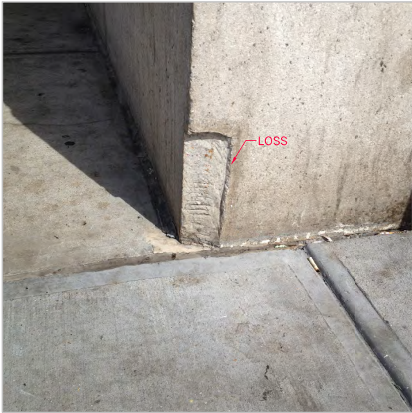
LOSS AT CORNER OF STONE UNIT
