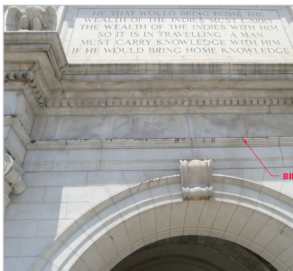
EVIDENCE OF WATER INFILTRATION AND LIQUID APPLIED BIRD REPELLENT AT MAIN PORTICO
