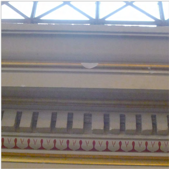
SPALL AT PLASTER CORNICE
