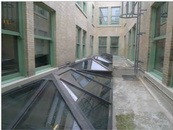
REPLACEMENT SKYLIGHTS AND ROOFING
