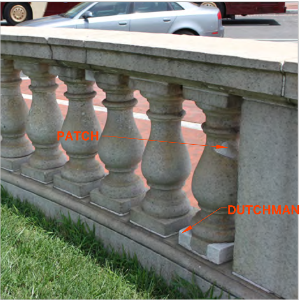
CRACKS AND PATCHES ON BALUSTERS
