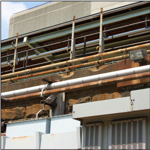
STRUCTURES INSTALLED NEAR WALL; HEAVY FERROUS STAINING
