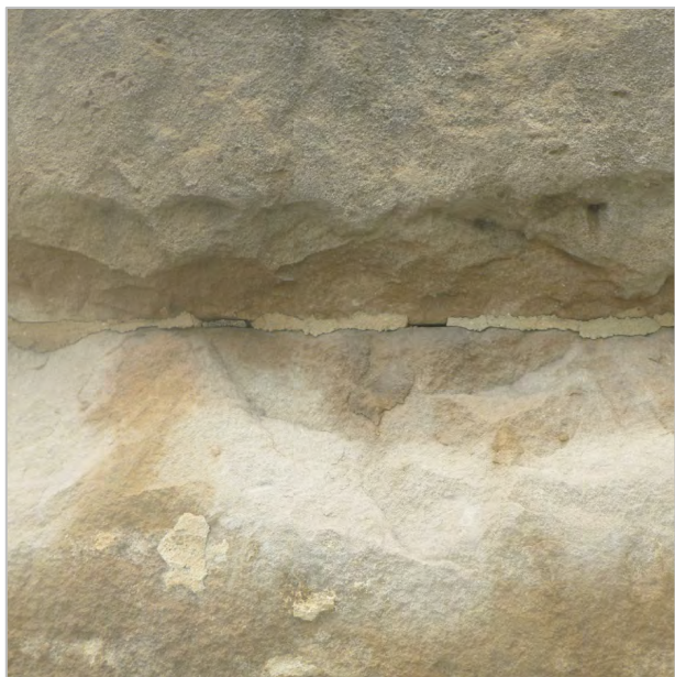
OPEN JOINT AT REBUILT STONE WALL
