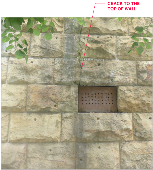
CONTINUOUS CRACK AT LINTEL
