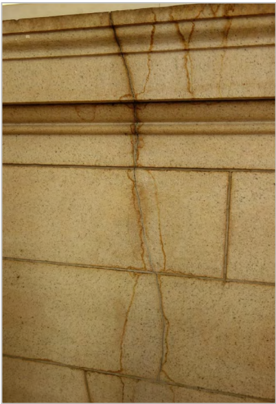
CONTINUOUS CRACK AND WATER STAIN
