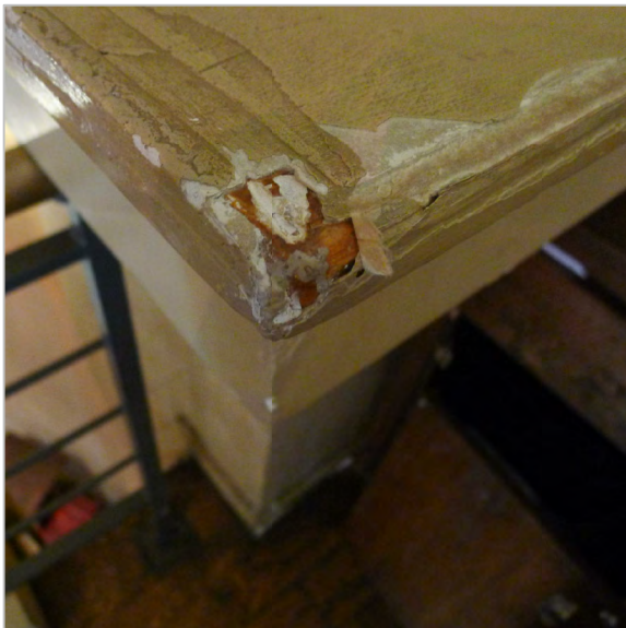
SPALL IN PLASTER
