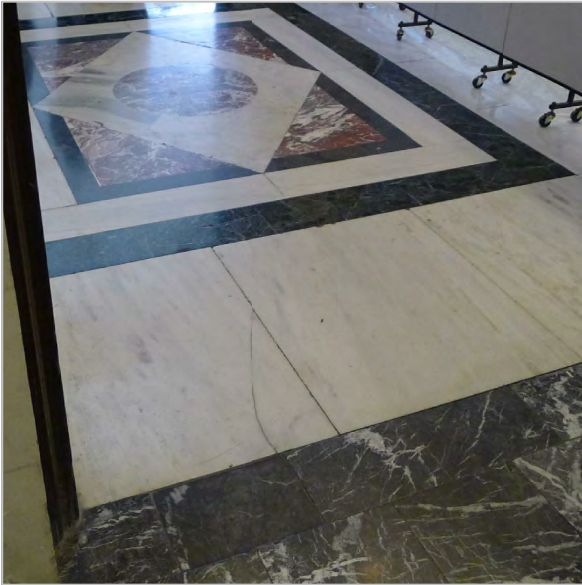
CRACK AT MARBLE FLOOR
