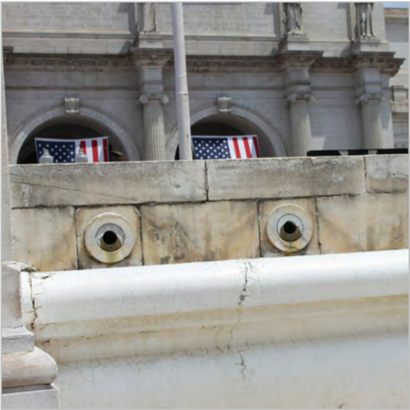
STAINING AND STONE DETERIORATION AT WATER SPOUT
