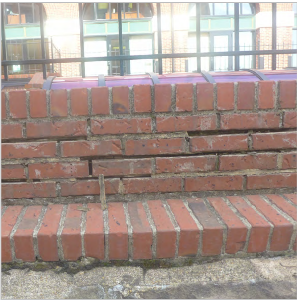
OPEN JOINTS AND LOOSE BRICKS
