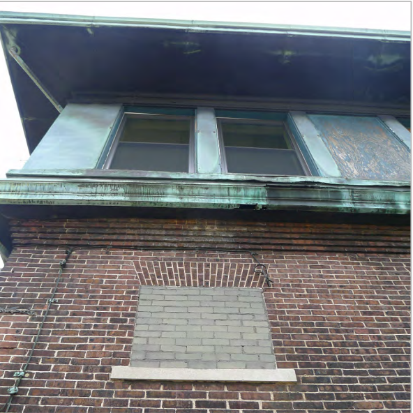
WATER STAINING AND BENT COPPER CLADDING
