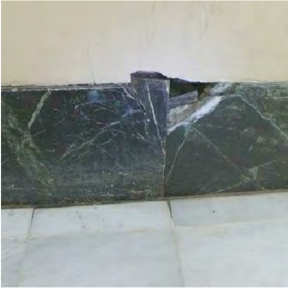
CRACKED, SPALLED, AND LOOSE MARBLE BASE
