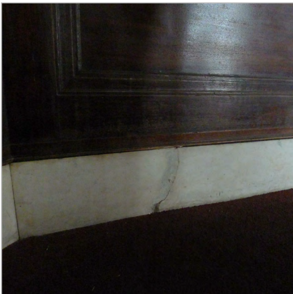
CRACK AT MARBLE BASEBOARD (EAST RETIRING ROOM)
