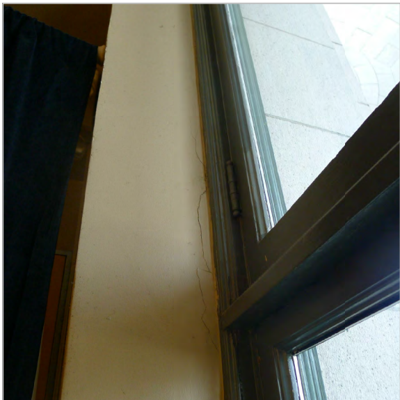
CRACK IN PLASTER
