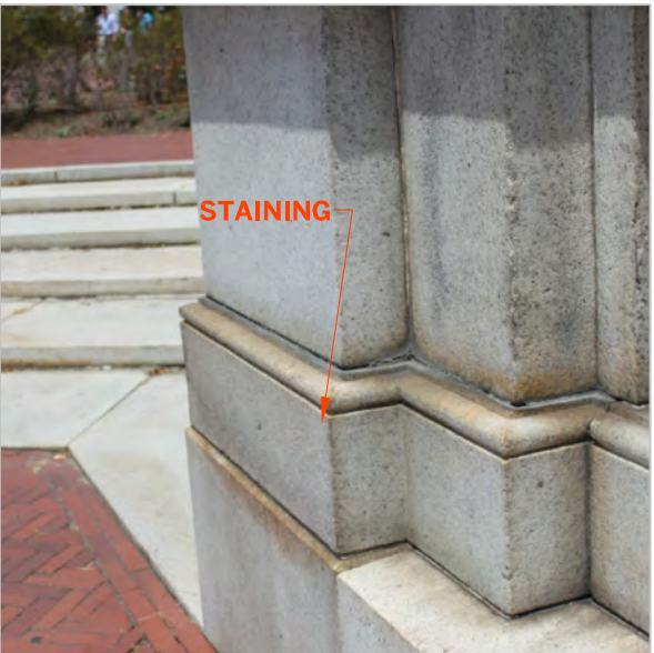
STAINING ON STONE BALUSTRADE
