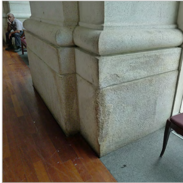
SURFACE LOSS AND SCALING
