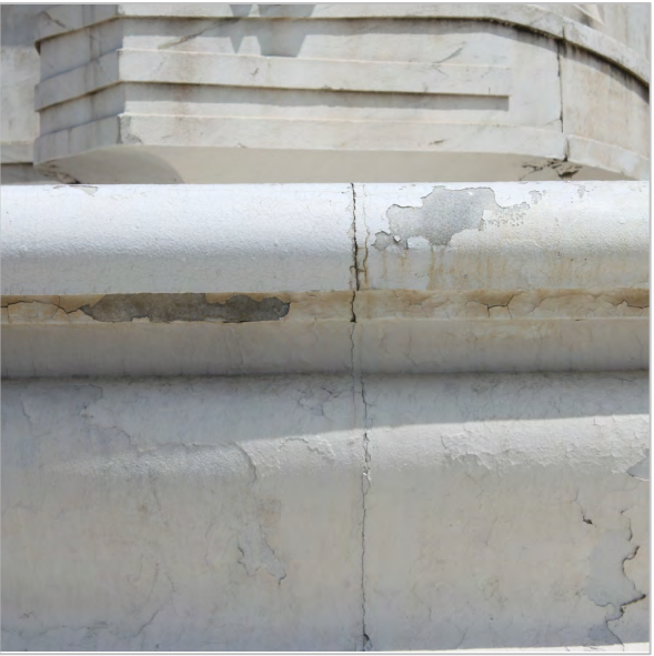
PAINT FAILURE ON FOUNTAIN BASIN
