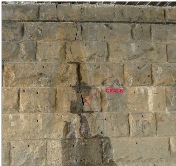
CONTINUOUS CRACK WITH WATER INFILTRATION AT FLORIDA AVENUE UNDERPASS
