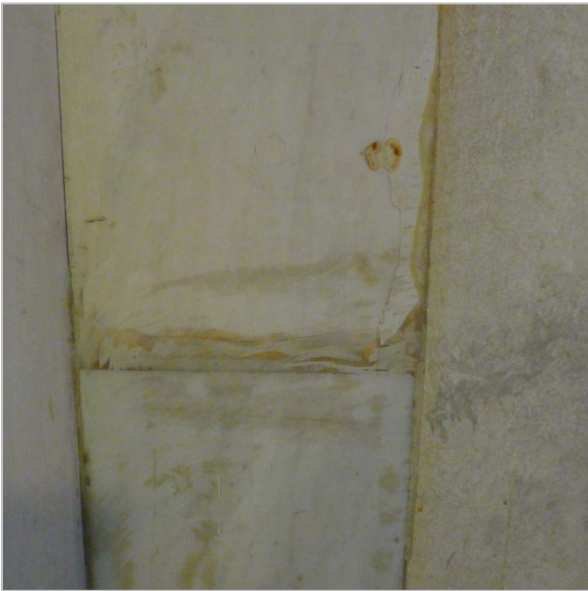
CRACKED AND LOOSE STONE
