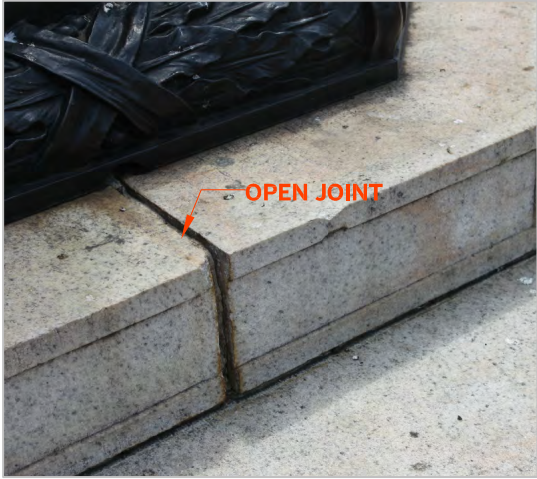
OPEN JOINTS IN GRANITE PEDESTAL
