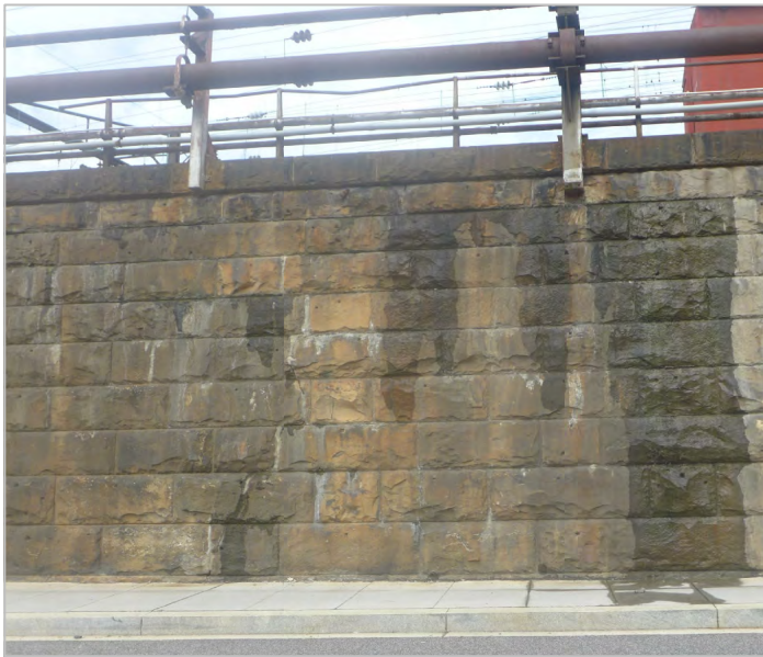
WATER INFILTRATION THROUGH WALL
