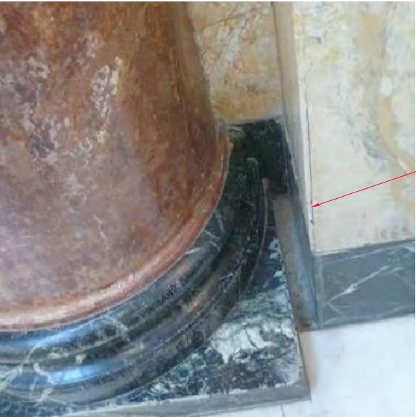
OPEN JOINT AT SCAGLIOLA PILASTER
