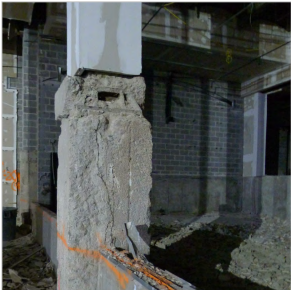
CRACKED COLUMN FOUNDATION
