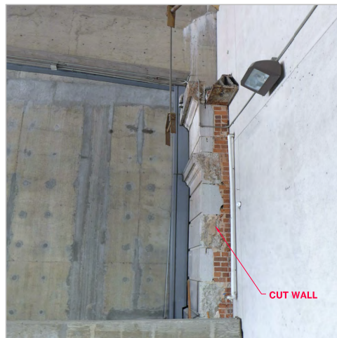
ORIGINAL MASONRY WALL CUT AT NEW RAMP, EAST CORNER
