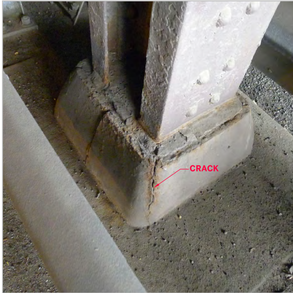
CRACKED COLUMN BASE AT FLORIDA AVENUE UNDERPASS
