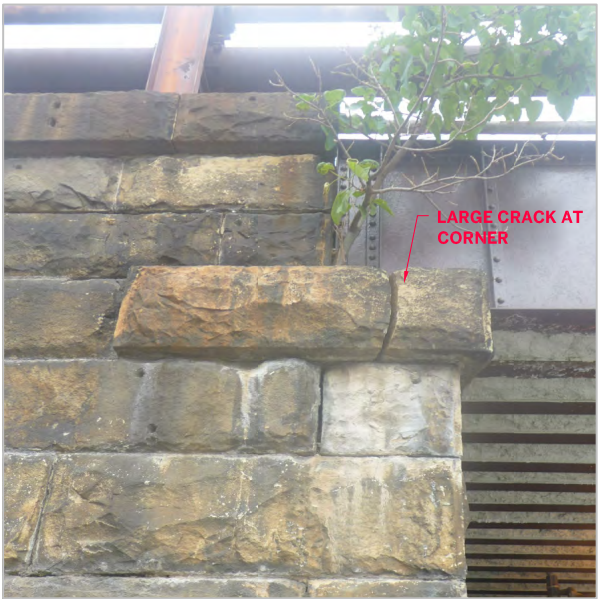
CRACKED CORNER STONE
