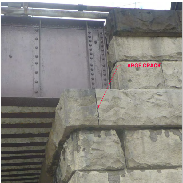
CRACK AT CORNER STONE UNIT
