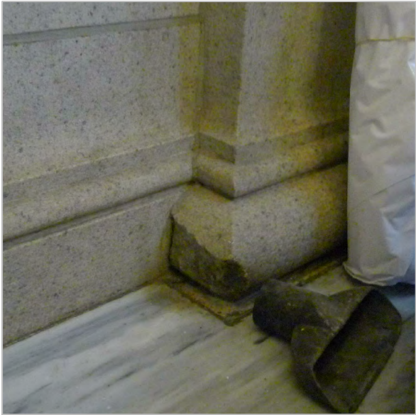
SPALL AT GRANITE BASE
