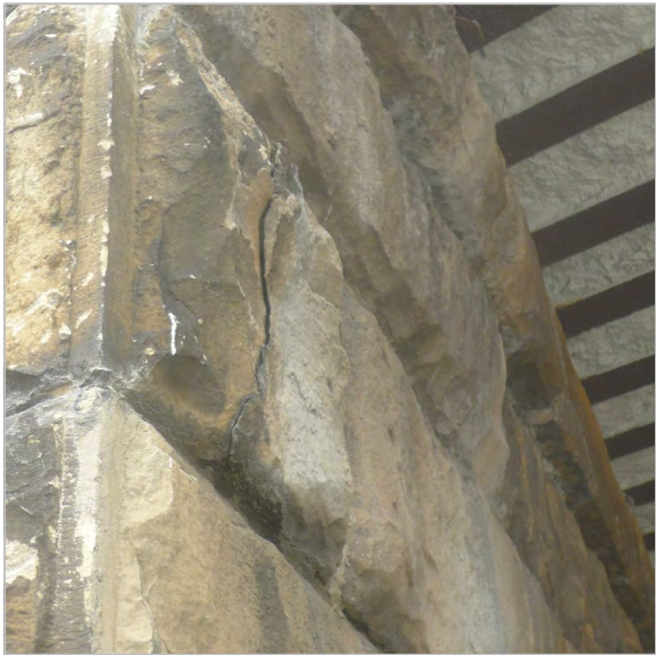
LOOSE SPALL AT M STREET UNDERPASS
