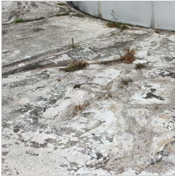
BASIN COATING FAILURE
