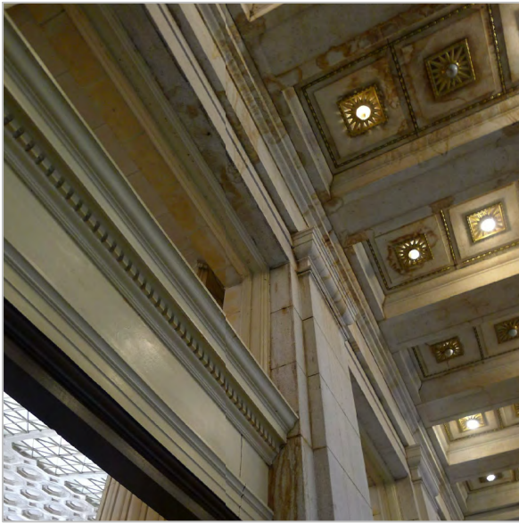
WATER-STAINED AND SOILED GRANITE CEILING AND WALL
