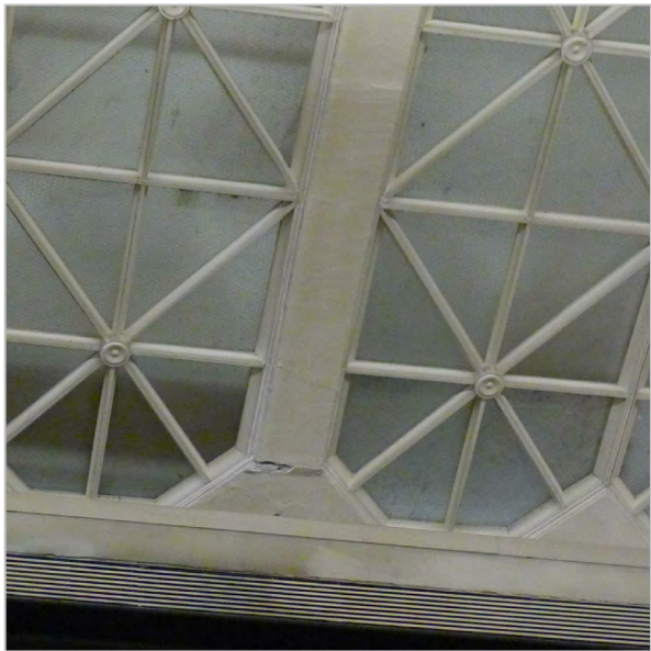
CRACK AT PLASTER BETWEEN LAYLIGHTS, TYP.
