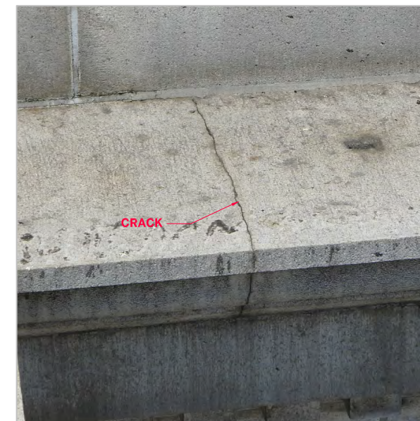
CRACK THROUGH CORNICE UNIT
