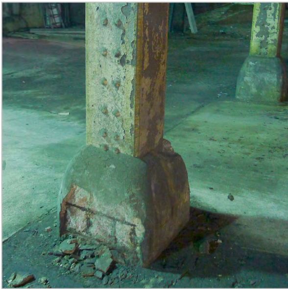
RUSTED COLUMN AND BROKEN CAST IRON BASE AT H STREET UNDERPASS
