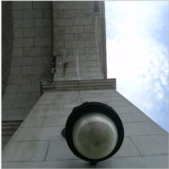
EVIDENCE OF WATER INFILTRATION AND STAINING AT ARCH
