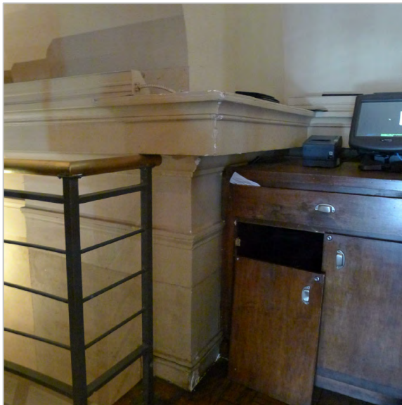
DAMAGED PLASTER CORNER
