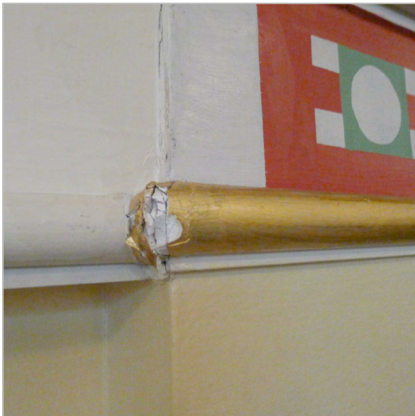
CRACK AND SPALL AT PLASTER CORNICE
