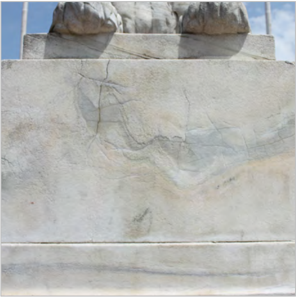
MAP CRACKING ON STONE SURFACE
