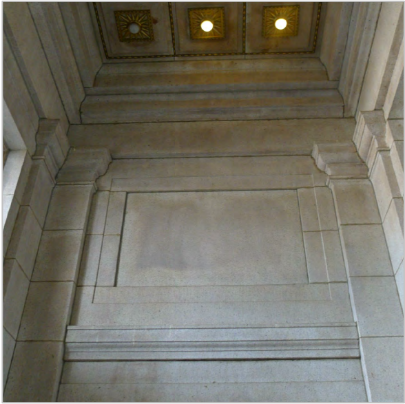
SOILED GRANITE CEILING AND WALL
