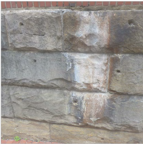
EFFLORESCENCE
