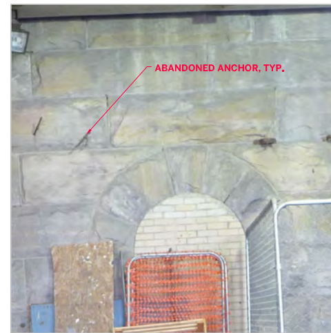
ABANDONED ANCHORS IN MASONRY WALL
