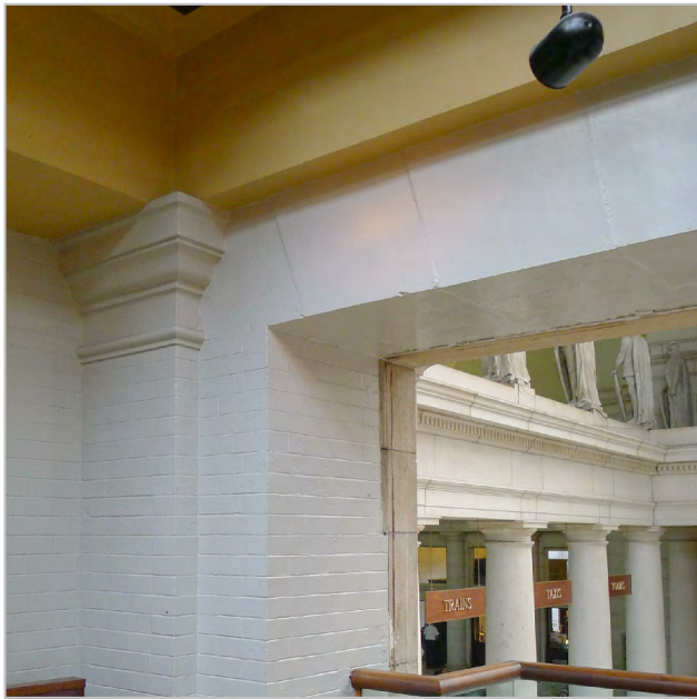
BRICK WALL AND TERRA COTTA LINTEL
