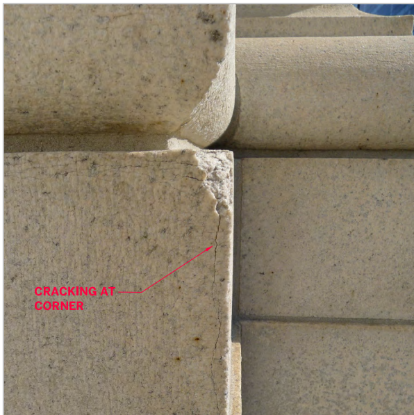
CRACKING AT CORNER OF GRANITE
