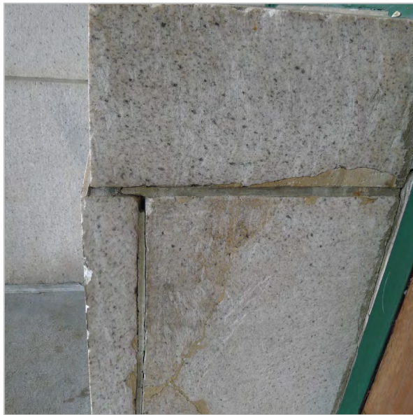
CRACKS AND SPALLS AT NON-ORIGINAL DOOR OPENING
