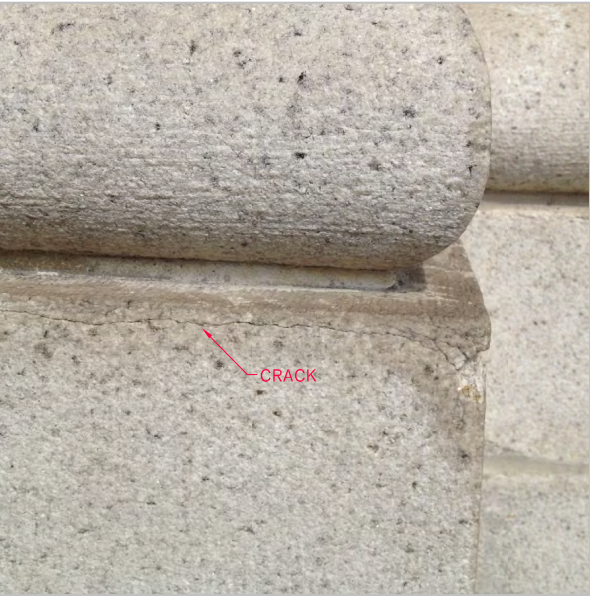
CONTINUOUS CRACK
