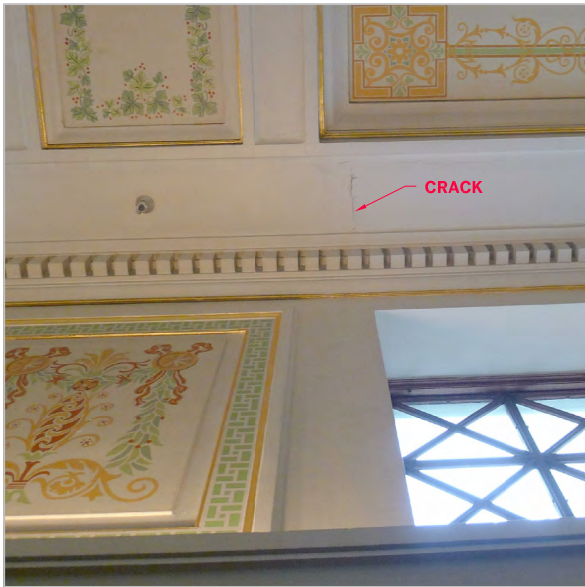
CRACKED PLASTER CEILING
