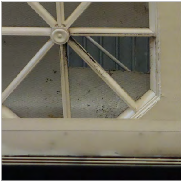
MISSING/BROKEN GLASS
