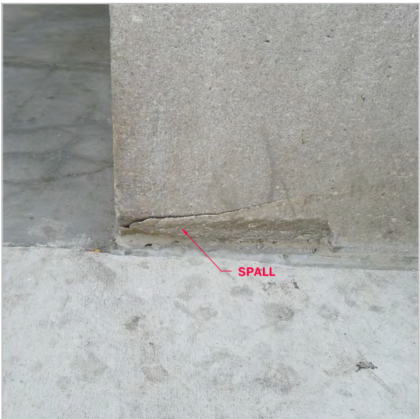
SPALL AT CORNER GRANITE UNIT
