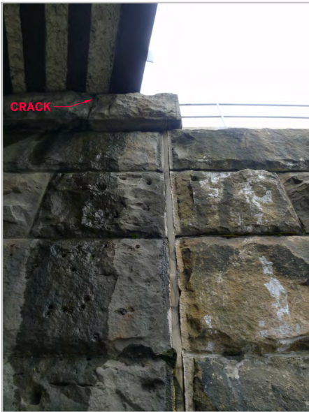
CRACKED STONE AND WATER INFILTRATION AT FLORIDA AVENUE UNDERPASS
