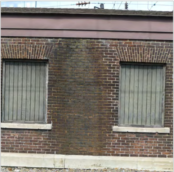
STAINING, SURFACE DAMAGE, MORTAR DETERIORATION, SPALLS
