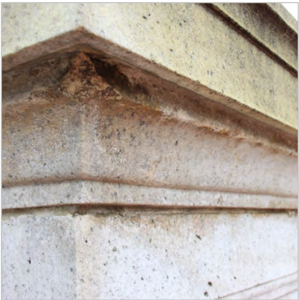
DISAGGREGATION OF GRANITE ON TOP RAIL OF BALUSTRADE
