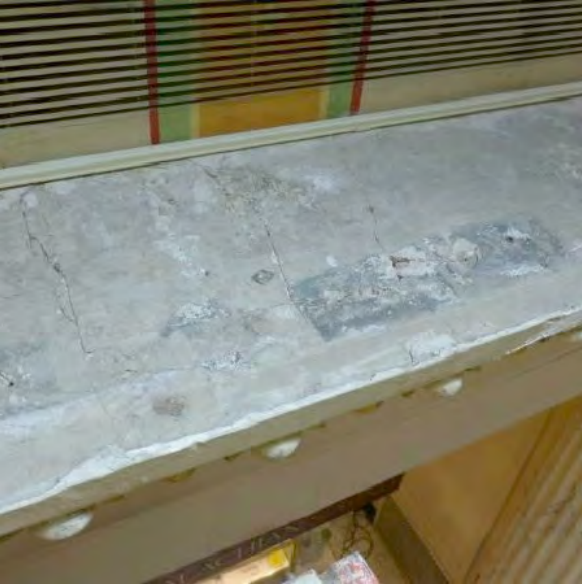
CRACKED LEDGE CLOSE TO ORIGINAL LIGHT COVE
