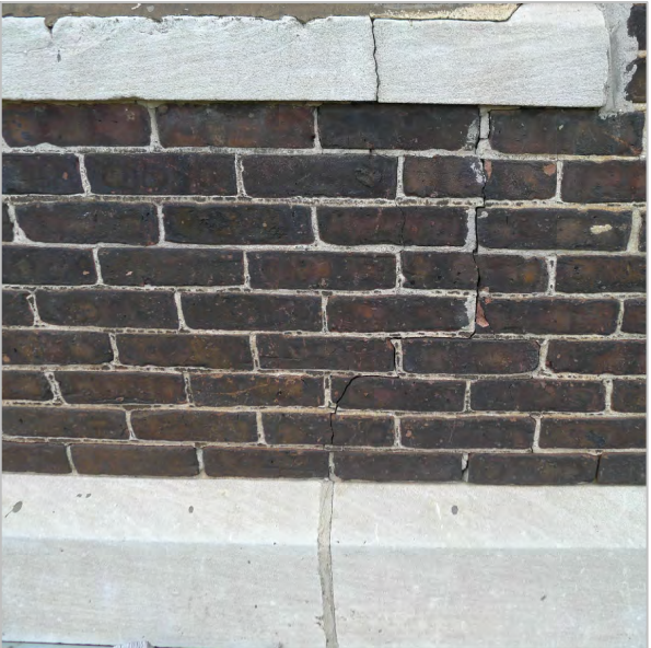
CONTINUOUS CRACK UNDER WINDOW
