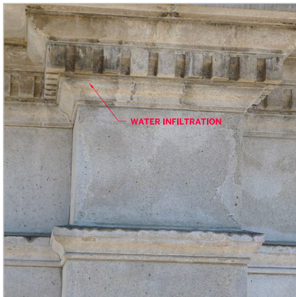
WATER INFILTRATION AT EAST SIDE
