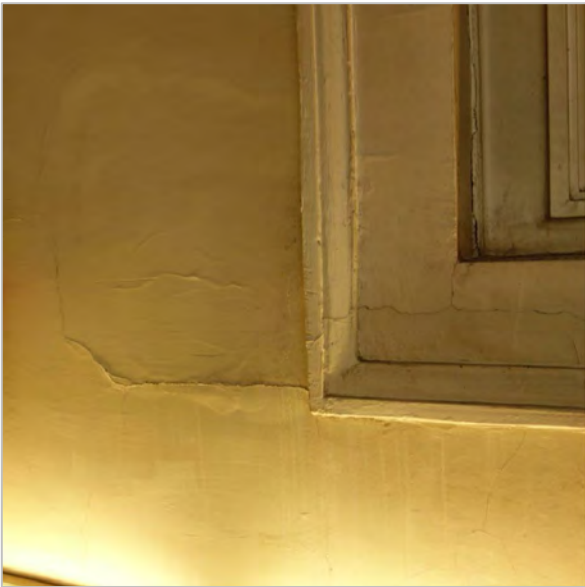
CRACKED PLASTER
