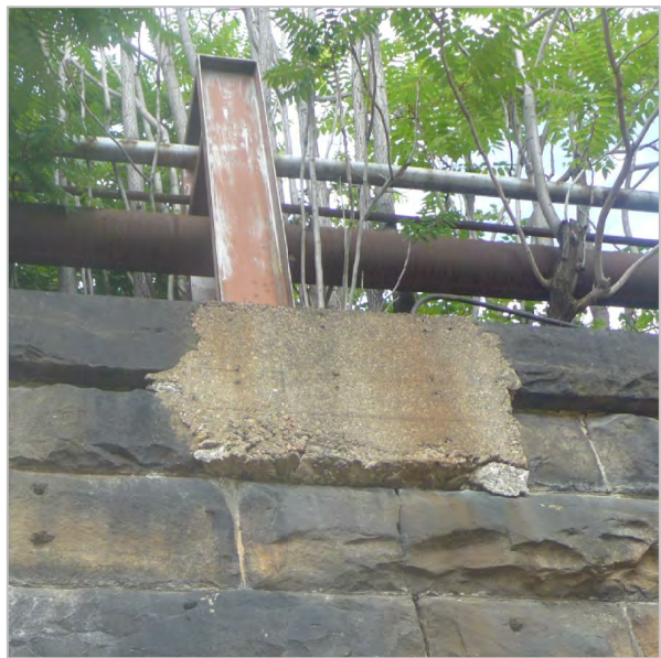
CONCRETE PATCH AT COPING
