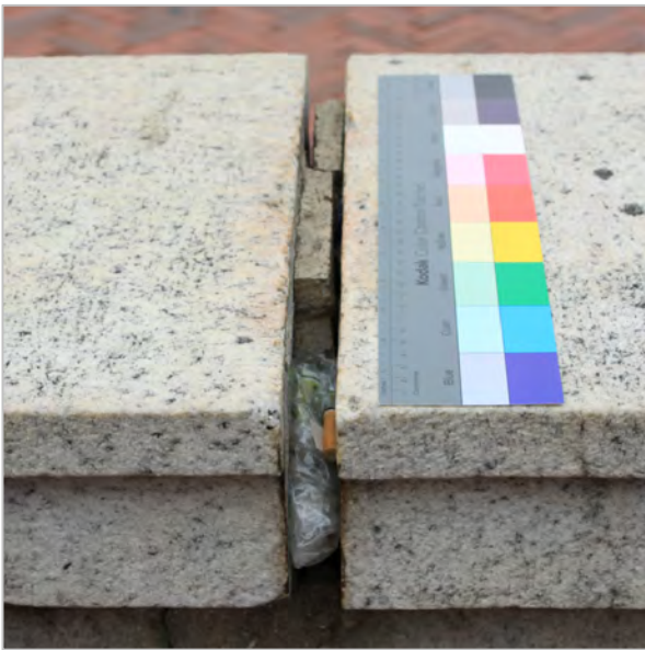
OPEN MORTAR JOINTS
