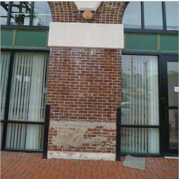
MORTAR RESIDUE
