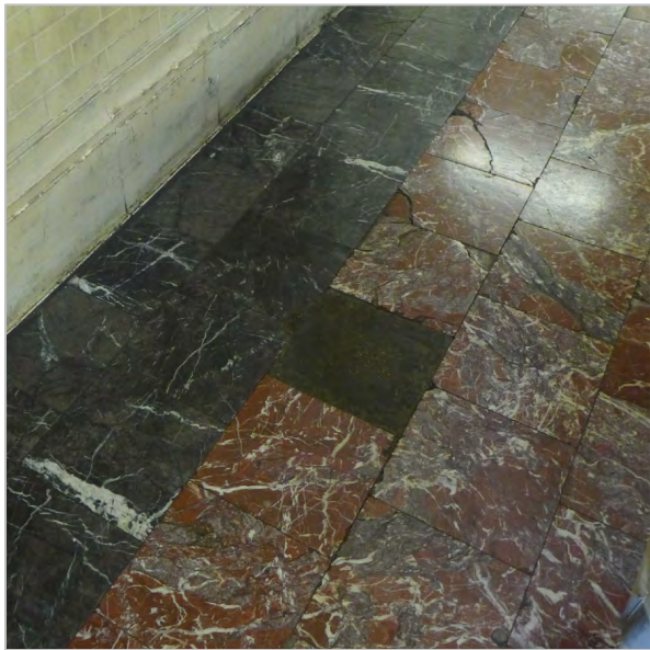
CRACKED AND DISPLACED MARBLE TILE FLOOR, TYP.
