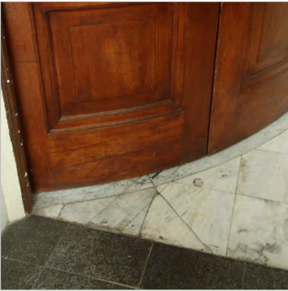
CRACK AT MARBLE FLOOR (SOUTH VESTIBULE)
