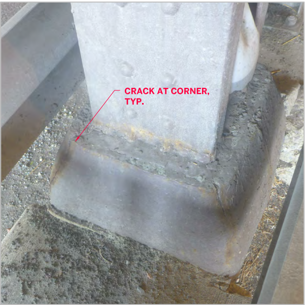
CRACKED CAST IRON COLUMN BASE AT I STREET UNDERPASS
