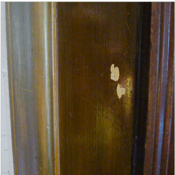
IMPACT AT PLASTER PANEL (EAST RETIRING ROOM)
