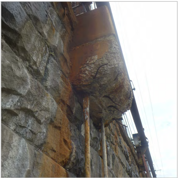
SPALLING CONCRETE
