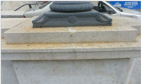
CRACK AT COPING
