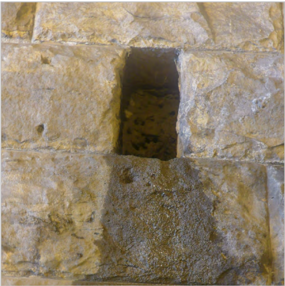
MISSING STONE AT K STREET UNDERPASS
