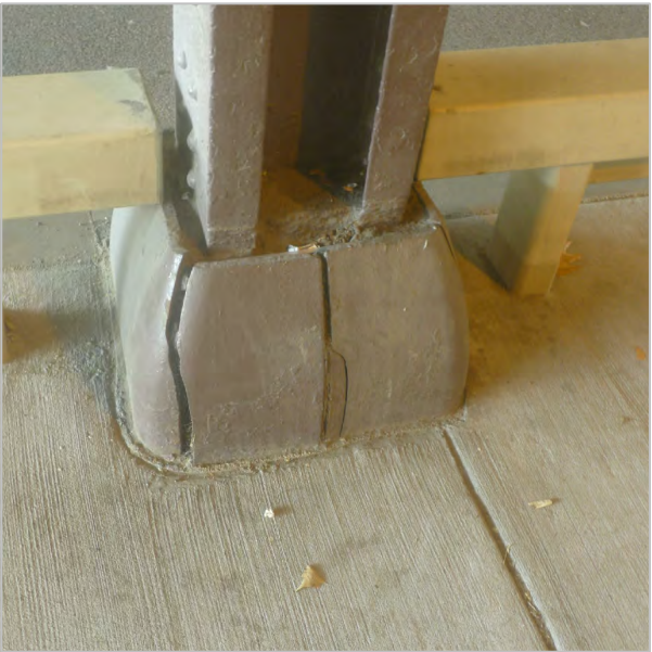
CRACKED CAST IRON COLUMN BASE AT M STREET UNDERPASS
