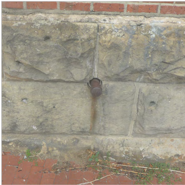
ABANDONED ANCHOR AT STONE WALL
