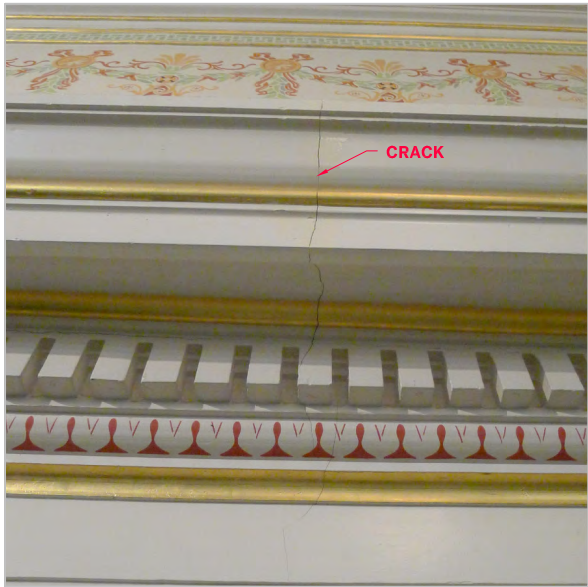
CRACK AT PLASTER CORNICE
