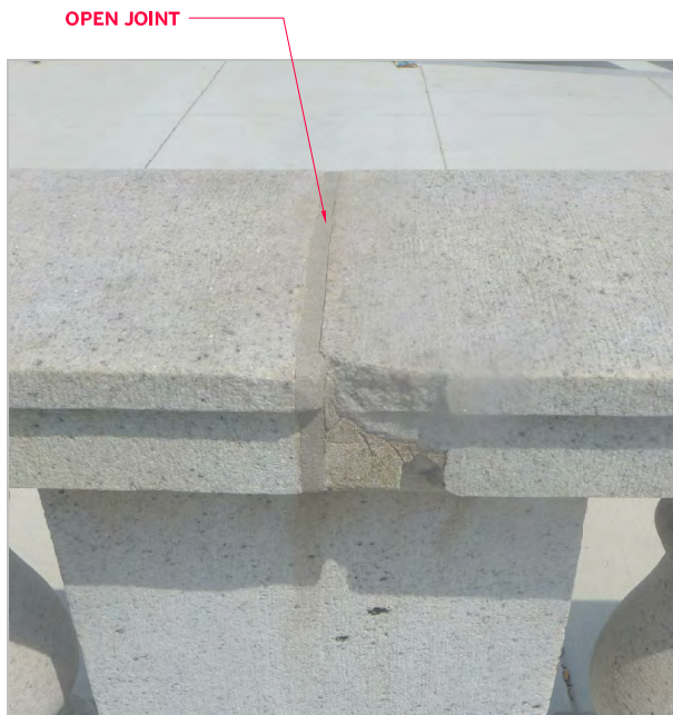
SPALL AND PATCH AT GRANITE
