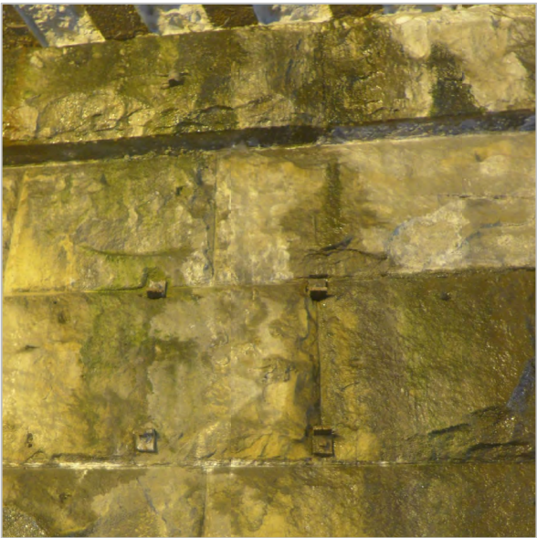
ABANDONED ANCHORS AT K STREET UNDERPASS
