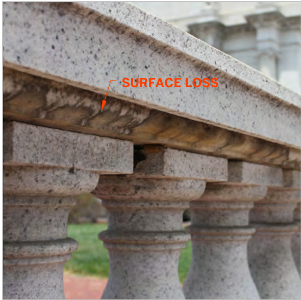
SURFACE LOSS AT UNDERSIDE OF RAILING
