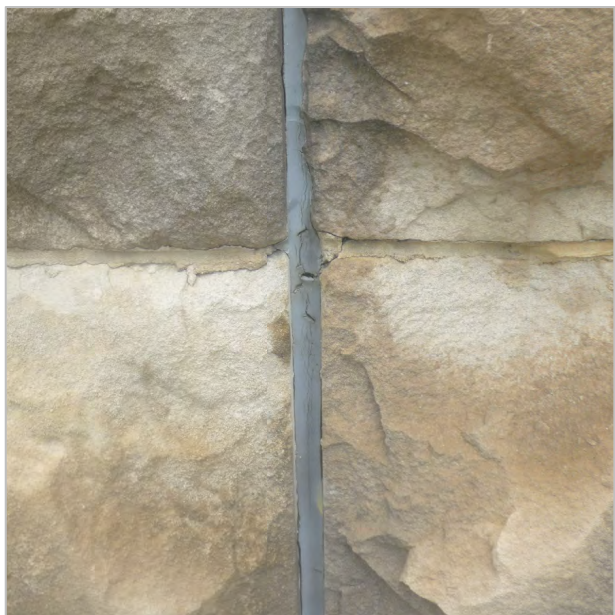
EXPANSION JOINT AT NEW WALLS
