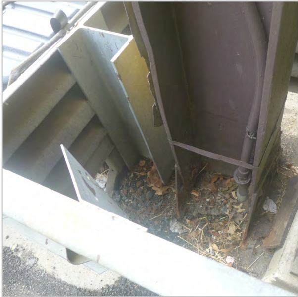
MISSING COLUMN BASE AT I STREET UNDERPASS
