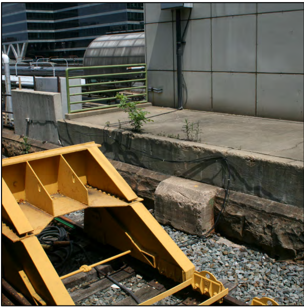
CONCRETE INFILL; FERROUS STAINING AND SOILING
