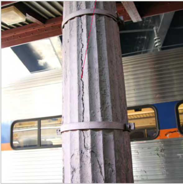
CRACKING THROUGH COLUMN
