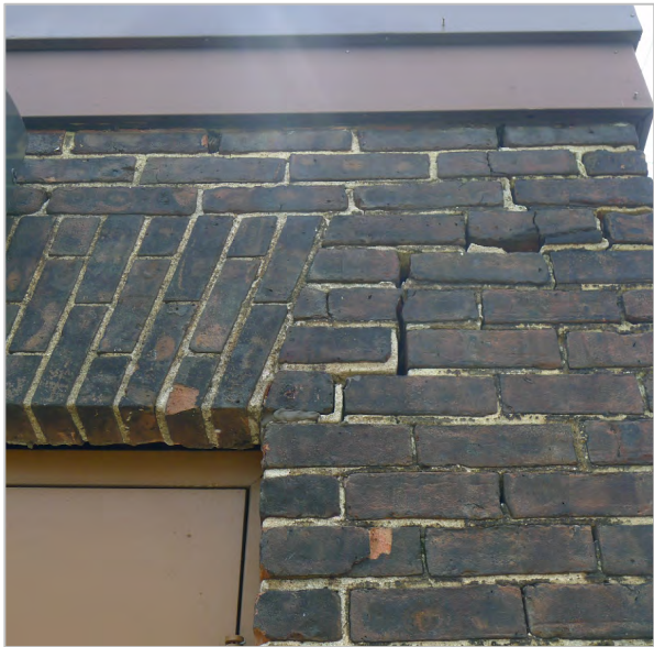
CONTINUOUS CRACK AT NORTH ELEVATION
