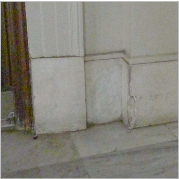
SPALL AT MARBLE BASEBOARD (SOUTH VESTIBULE)
