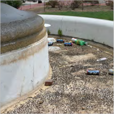
EXPOSED CONCRETE IN BASIN
