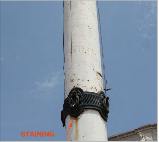
PAINT FAILURE ON FLAGPOLE SHAFT
