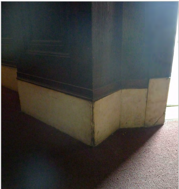
SPALLS AT MARBLE BASEBOARD (EAST RETIRING ROOM)
