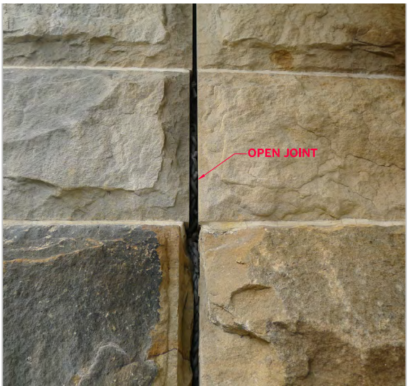
OPEN JOINT BETWEEN NON-HISTORIC AND ORIGINAL WALL AT FLORIDA AVENUE UNDERPASS
