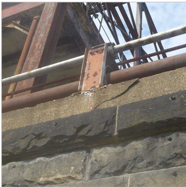
SPALLED CONCRETE COPING
