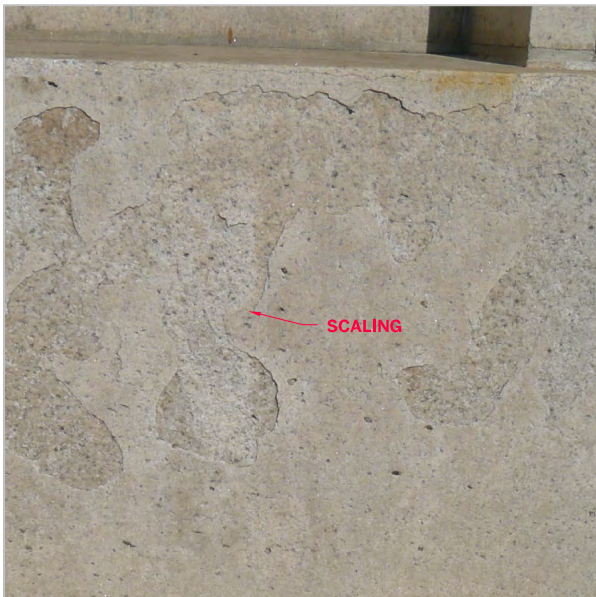
SCALING AT BASE OF GRANITE WALL
