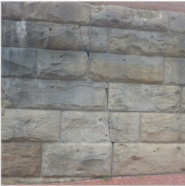
CONTINUOUS CRACK
