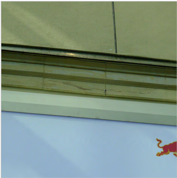
CRACKED AND DISPLACED PIECES AT TERRA COTTA CORNICE (FORMER NORTH EXTERIOR WALL)
