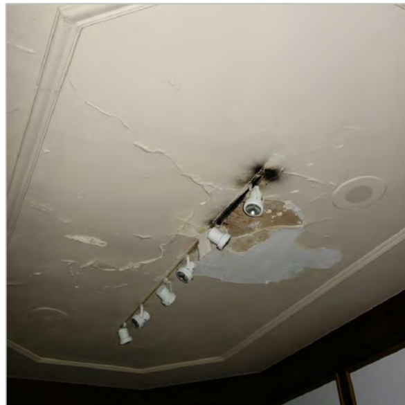
PLASTER CEILING WATER DAMAGE (WEST RETIRING ROOM)
