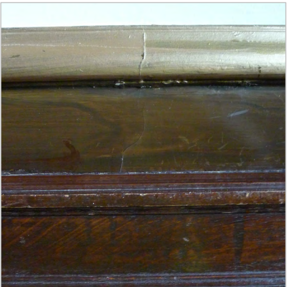
CRACKED PLASTER MOLDING (EAST RETIRING ROOM)
