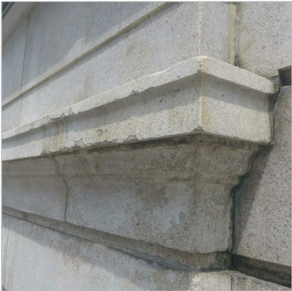
SCALING AND SPALLING GRANITE
