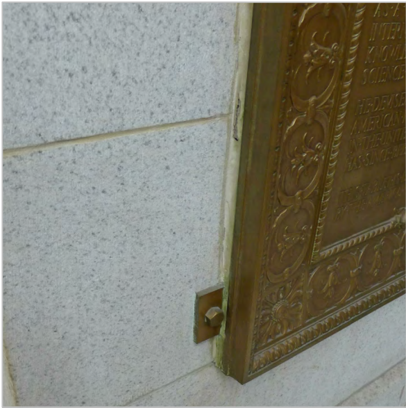
OPEN JOINT AROUND PLAQUE
