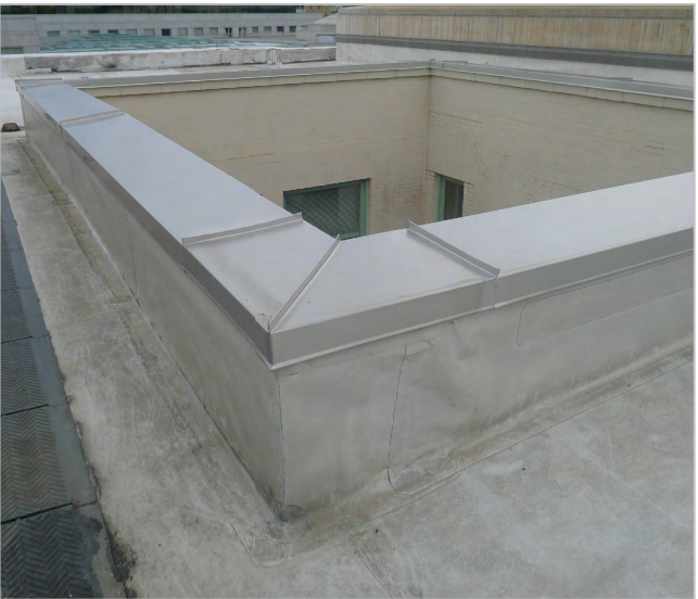
REPLACEMENT ROOFING MATERIAL AND FLASHING
