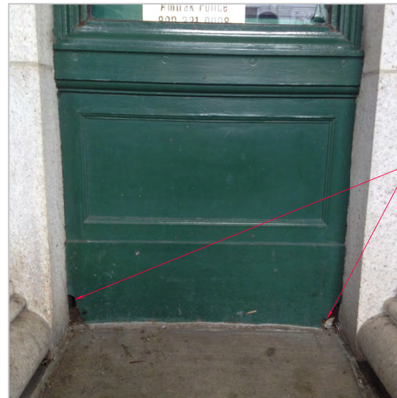
LOSS AT CORNERS OF WINDOW FRAME
