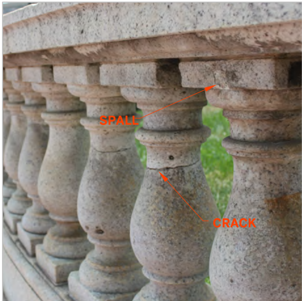
SPALLS AND CRACKS AT BALUSTERS
