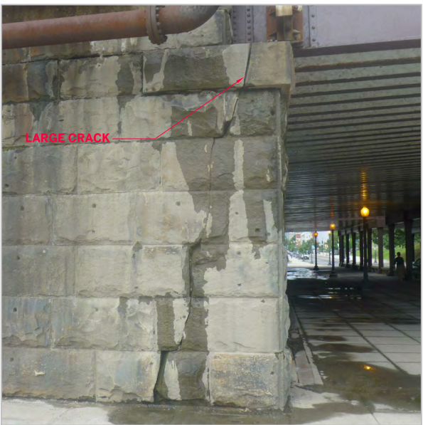
CONTINUOUS CRACK AT WALL CORNER
