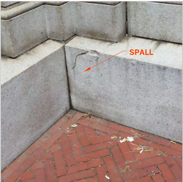
SPALL AT BASE OF BALUSTRADE
