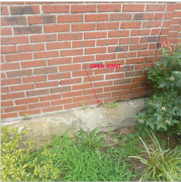
OPEN JOINT BETWEEN STONE AND BRICK
