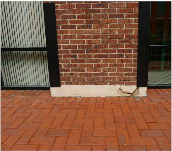
SPALLS AT STONE BASE
