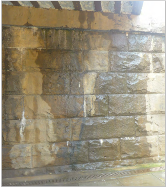
CONTINUOUS CRACK AT I STREET UNDERPASS
