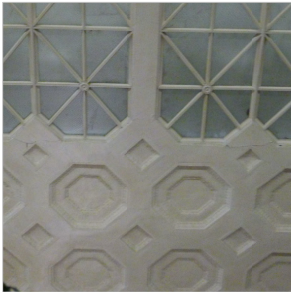
CRACK AT PLASTER
