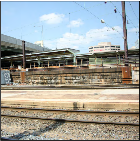
FERROUS STAINING
