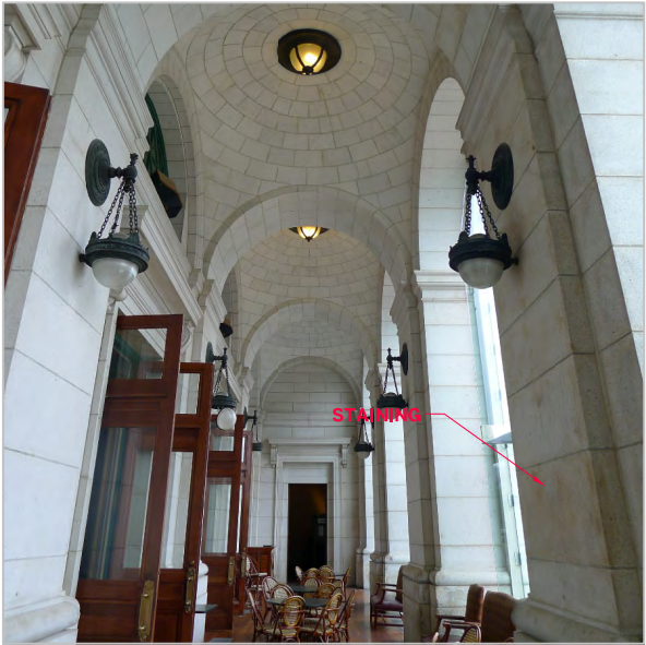
STAINING AT EAST WALL UNDER CEILING
