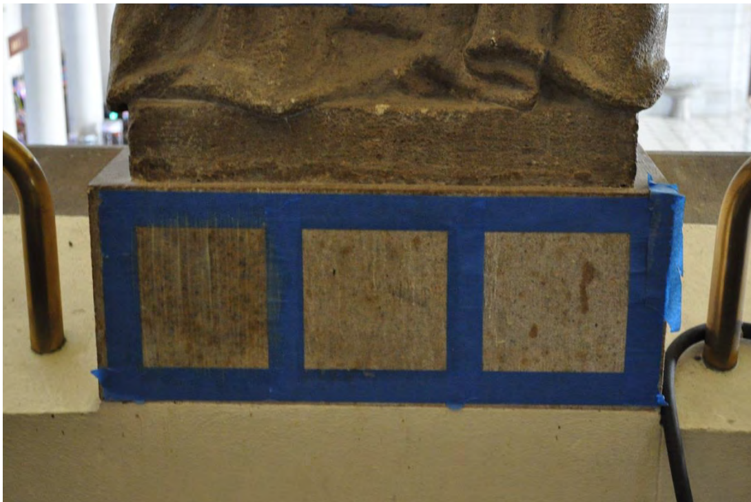
Figure 13. Mockups after poultice removal. L-R MasonRE, Dri-Klean, & dry soot sponge.
