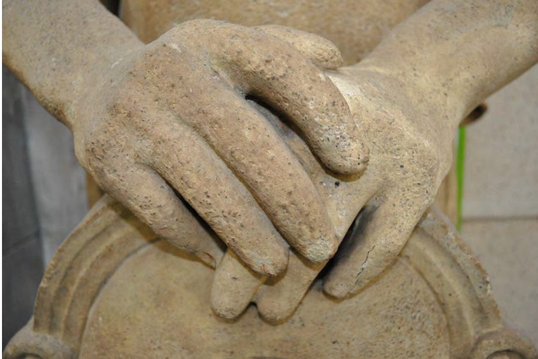
Figure 8. Cracks in Fingers.
