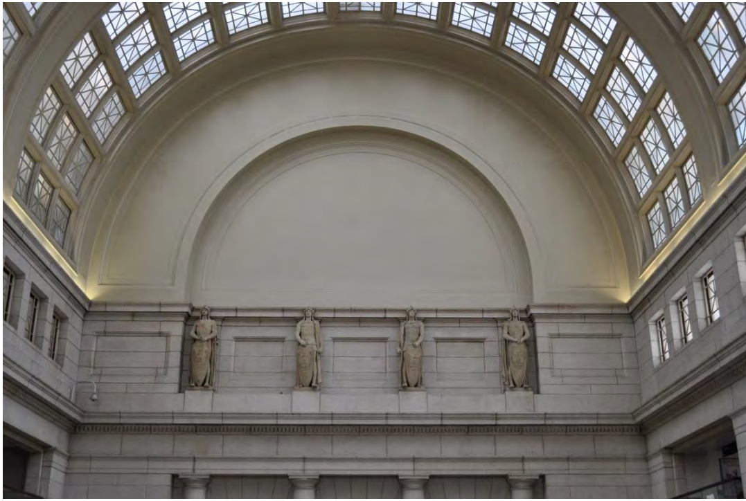
Figure 1. Prior to Restoration.
