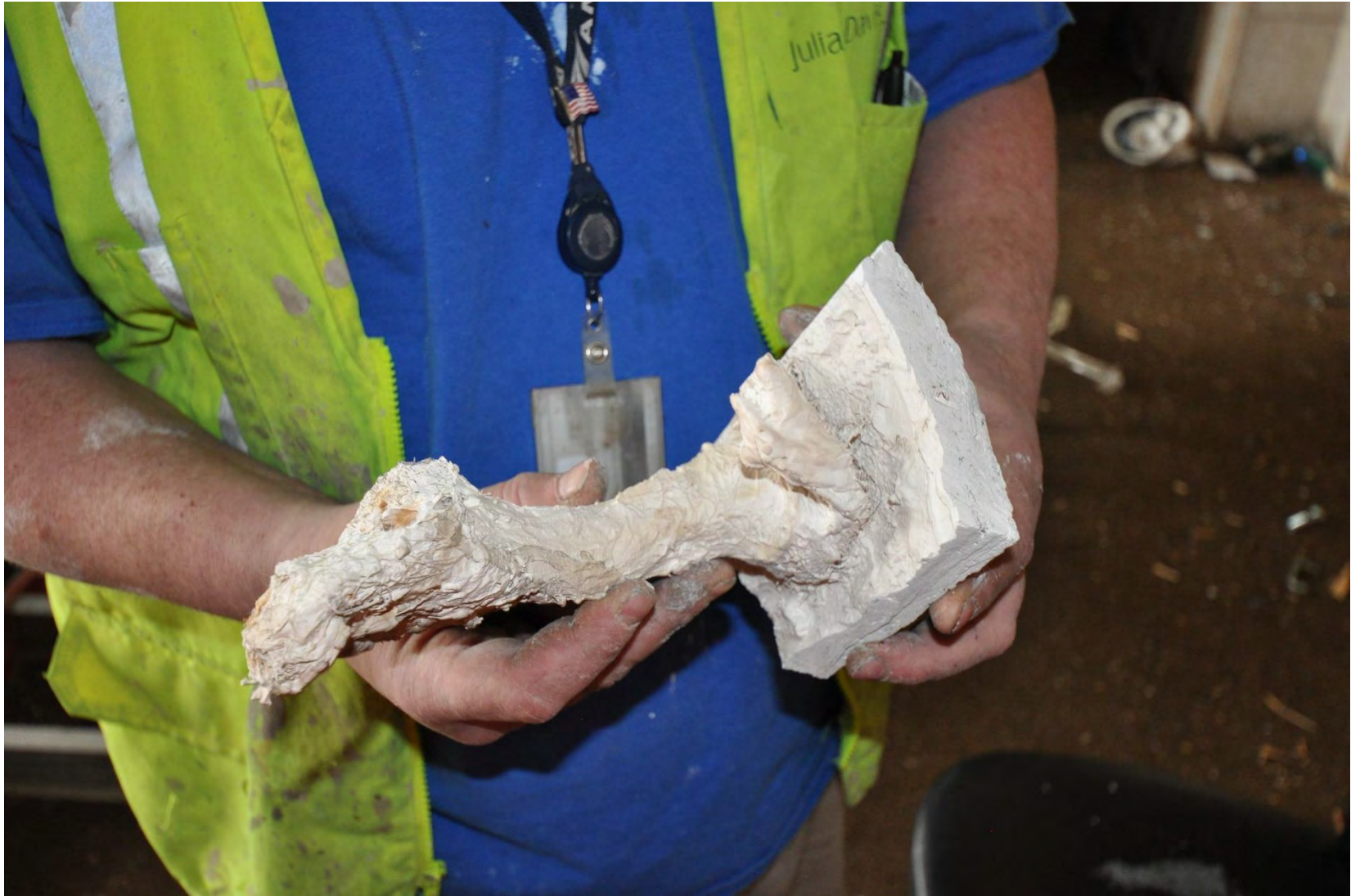
Examining the section that was sampled in 2016 for plaster analysis.
