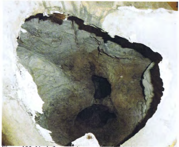
Figure 133. Neck flange prior to re-installation.
