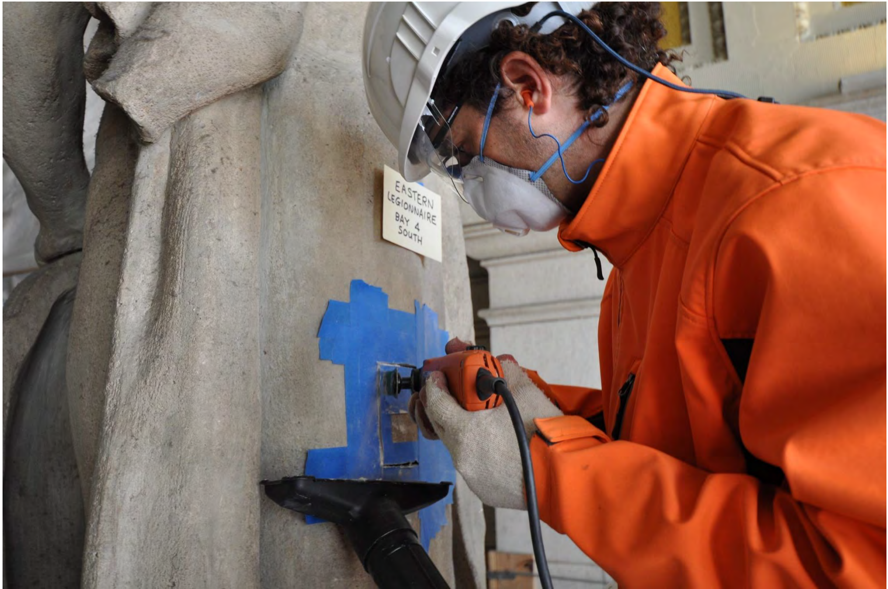
Worker carefully removing a section on the back of the statue as part of the 2016 plaster analysis.
