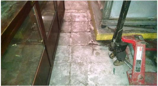
Photo 2. Homogeneous area HA2, grayish 12"x12" floor tile with mastic. 14.6% Chrysotile – Floor Tile; 3.8% Chrysotile - Mastic.
