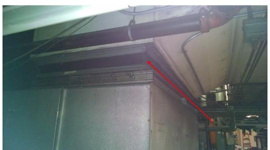
**Photo 4.** Homogeneous area HA3, black HV/AC vibration dampener. Presumed asbestos containing material.
