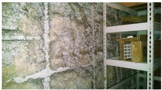
**Photo 1.** Homogeneous Area 1 (HA1), spray-on fireproofing. Asbestos not detected.
